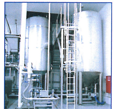
Like the kneading system also the pre-dough plant works continuously.
